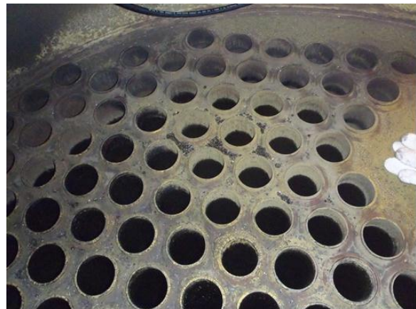
Pic 5 & 6: Top tube plate for economizer 1 with slight amounts of soot.
