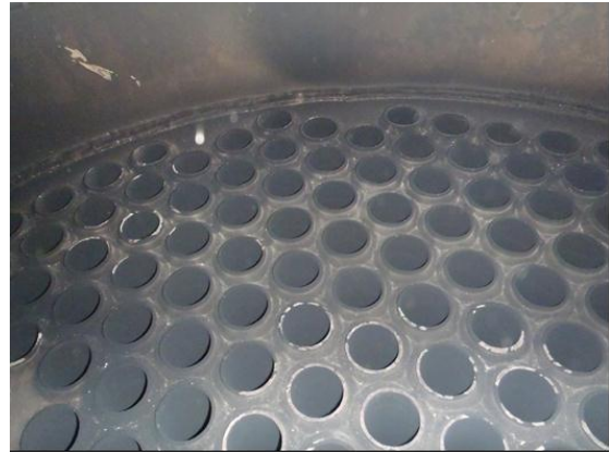
Pic 8 & 9: Top tube plate for economizer 2 with thick amounts of soot.
