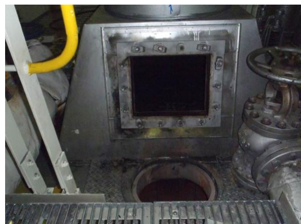
Pic no 1 & 2 Access to the furnace room and uptake space + manhole on top going to water space are open for entry.
