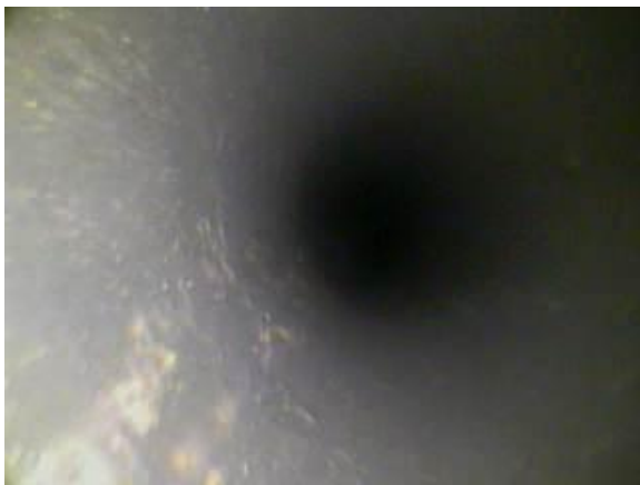
Pic 3: Tube 008- observed minor scaling
