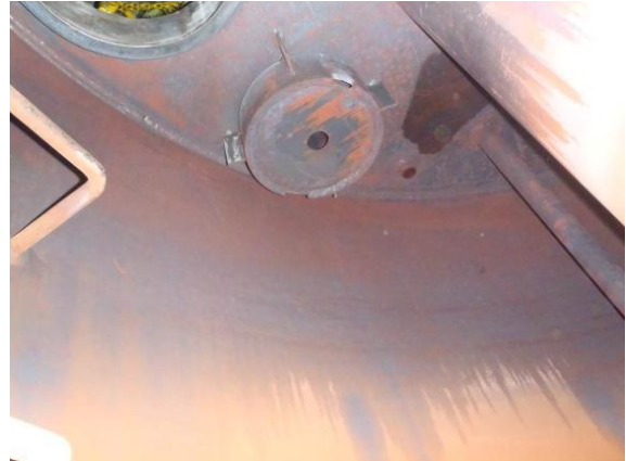
Pic no 20 & 21: Water side shell, top tube plate (Steam space) penetration piping were observed with no visible defects.
