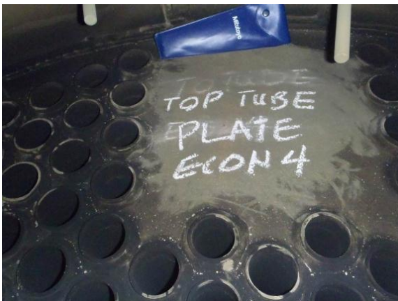
Pic 16 & 17: Top tube plate for economizer 4 with thick amounts of soot.
