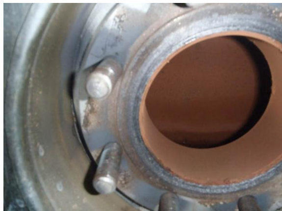
Pic no 16 & 17: Hand-hole No.01 & 3 seating in acceptable condition with small amounts of soot deposits noticed
