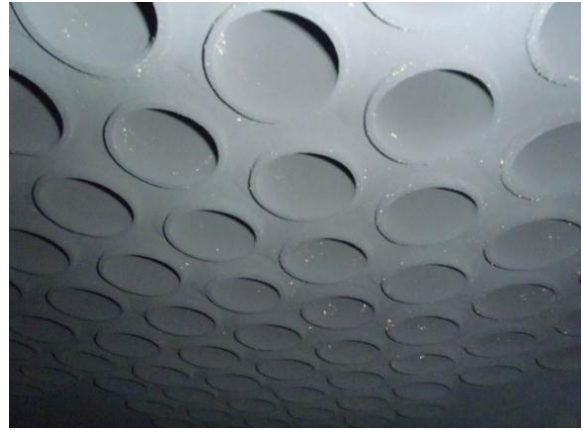
Pic 14 & 15: Top tube plate for economizer 3 with thick amounts of soot.
