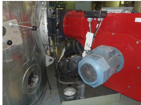
Pic no. 1 & 2: Burner opened for entrance. Area around the burner and full system appear to be in good clean condition.
