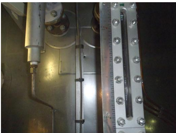
Pic 5 & 6 : Gauge glass found to be good condition with water visible and no signs of crack, mounting on top of boiler found to be in good condition.
