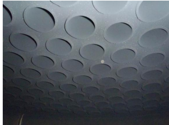
Pic 10 & 11: Top tube plate for economizer 2 with thick amounts of soot.
