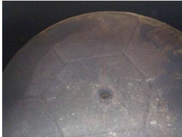
Pic no 5: Furnace entrance and furnace floor refractory
