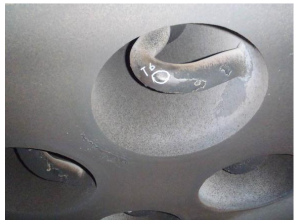
Pic no 6 & 7: Furnace shell plate with no sign deformation or buckle and pin element found to be in good condition, no visible crack or sign of leaked. Soot deposits in acceptable level.
