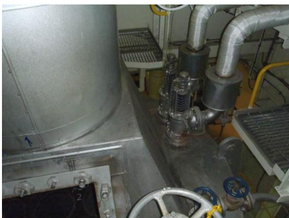
Pic no 3 & 4: Safety valves are in good condition outside and hand hole No.2 was found with minor sign of smoke (gas leak)
