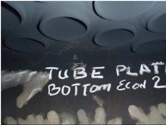
Pic 10 & 11: Top tube plate for economizer 2 with thick amounts of soot.
