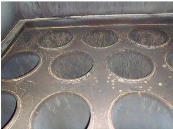
Pic 9: Tubes in gas uptake side in good condition
