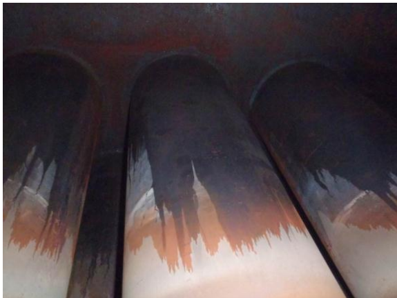
Pic no 24 & 25: Viewing the boiler steam space, pin tubes were found in very good condition. No internal corrosion and deposits found. End of auxiliary boiler no.1
