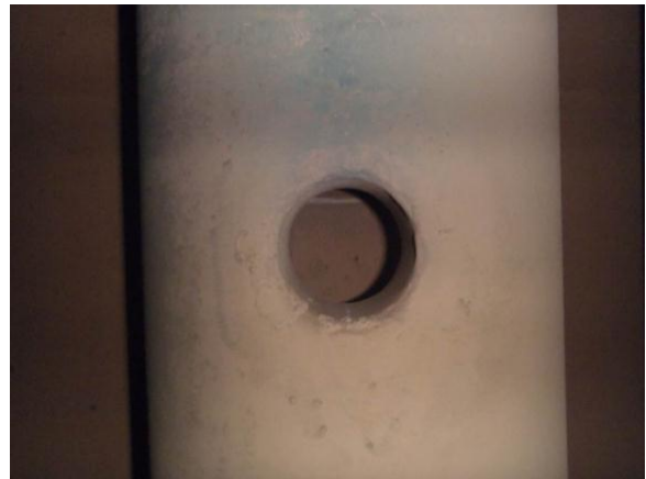
Pic no 24 & 25: Viewing the boiler steam space, pin tubes were found in very good condition. No internal corrosion and deposits found. End of auxiliary boiler no.1
