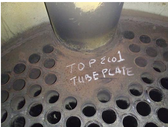
Pic 5 & 6: Top tube plate for economizer 1 with slight amounts of soot.
