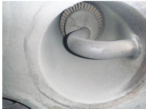
Pic 13 & 14: Bottom tube plate found without distortion and lower elbow of the pin element-weld connection has no visible crack
