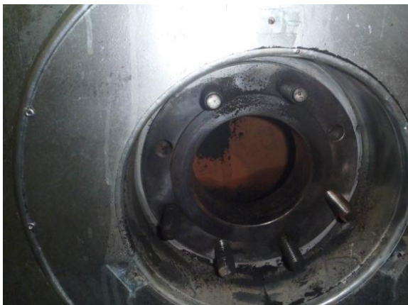
Pic no 16 & 17: Hand-hole No.01 & 3 seating in acceptable condition with small amounts of soot deposits noticed
