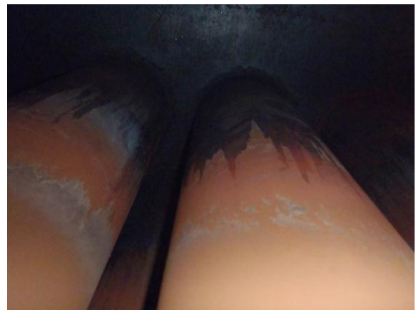
Pic no 11 & 12: Minors scales but not alarming found around the outlet hole some pin tubes
