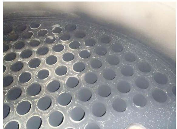
Pic 16 & 17: Top tube plate for economizer 4 with thick amounts of soot.
