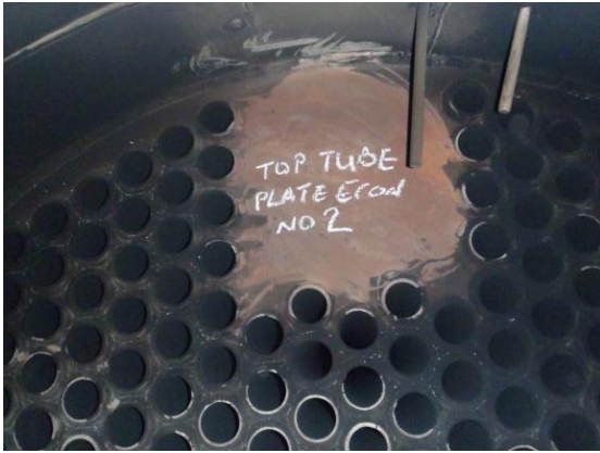
Pic 8 & 9: Top tube plate for economizer 2 with thick amounts of soot.
