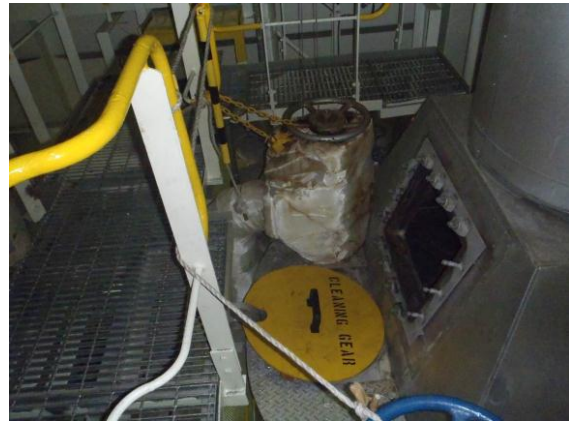
Pic 8: Entrance into the gas uptake and water side
