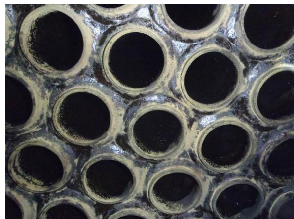
Pic 7 & 8: Top tube plate for economizer 2 with thick amounts of soot.
