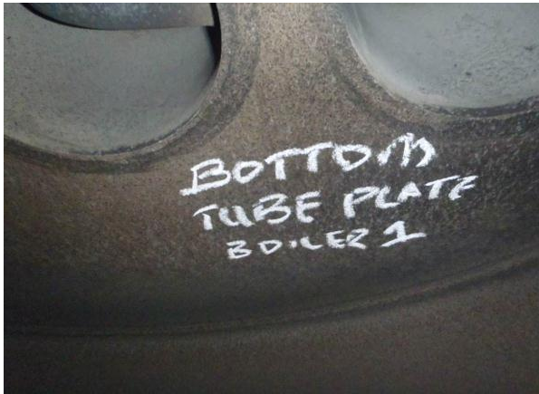
Pic 13 & 14: Bottom tube plate found without distortion and lower elbow of the pin element-weld connection has no visible crack
