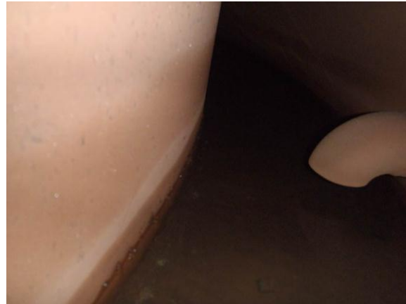
Pic no 18 & 19: Showing the bottom ring plate & furnace shell water side seen from hand hole No.1 & 3 respectively. No internal corrosion and negligible loose debris at the bottom
