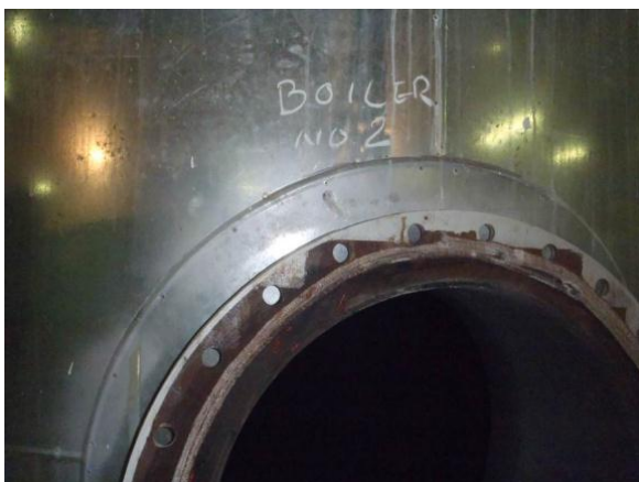
Pic no 1 & 2 Access to the furnace room and uptake space + manhole on top going to water space are open for entry.
