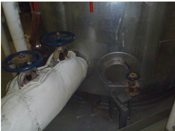
Pic no. 3 & 4: Valves in pillows, hand hole cladding, Water level gauge glasses and mountings still in acceptable condition.
