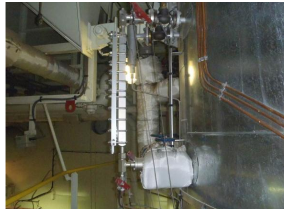
Pic no. 3 & 4: Valves in pillows, hand hole cladding, Water level gauge glasses and mountings still in acceptable condition.
