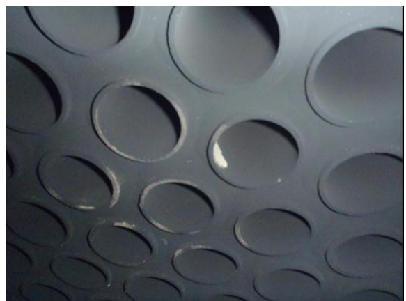
Pic 18 & 19: Top tube plate for economizer 4 with thick amounts of soot
