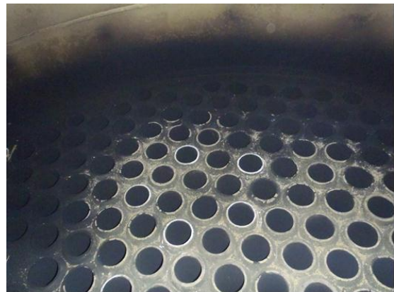
Pic 12 & 13: Top tube plate for economizer 3 with thick amounts of soot.
