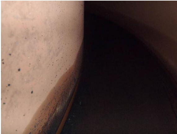
Pic no 18 & 19: Showing the bottom ring plate & furnace shell water side seen from hand hole No.1 & 3 respectively. No internal corrosion and negligible loose debris at the bottom
