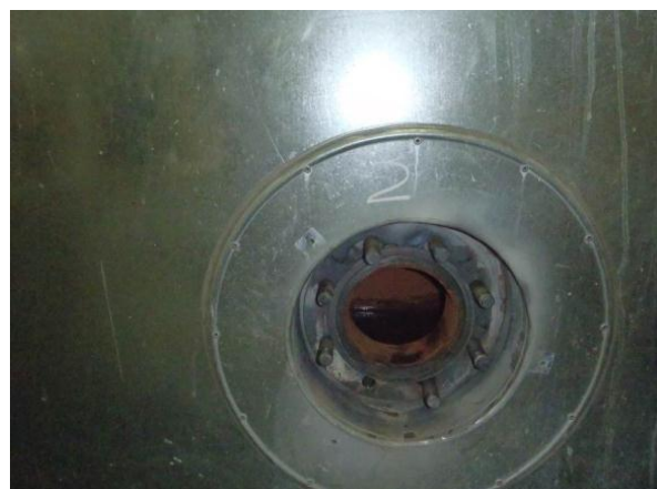
Pic no 3 & 4: Safety valves are in good condition outside and hand hole No.2 was found with minor sign of smoke (gas leak)
