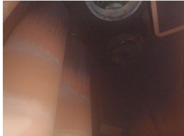
Pic no 9 & 10: Boiler shell plate was found in very good condition and the steam space the top tube plate, pin tubes were also found in good condition.
