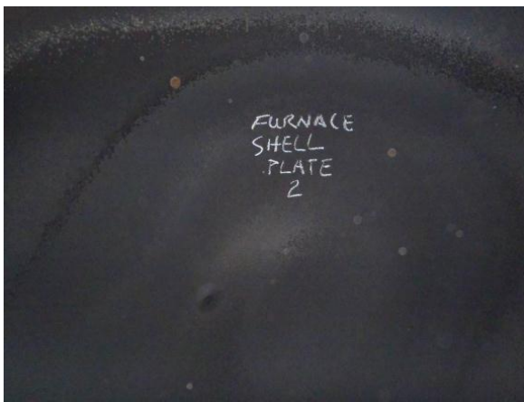
Pic no 6 & 7: Furnace shell plate with no sign deformation or buckle and pin element found to be in good condition, no visible crack or sign of leaked. Soot deposits in acceptable level.
