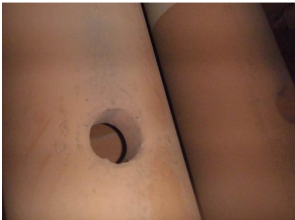
Pic no 11 & 12: Minors scales but not alarming found around the outlet hole some pin tubes
