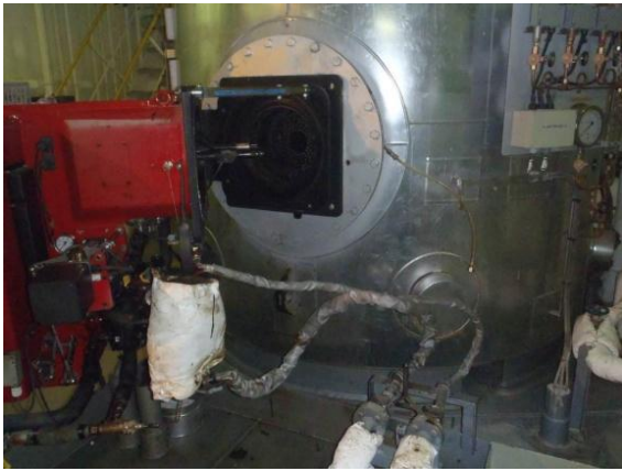
Pic no. 1 & 2: Burner opened for entrance. Area around the burner and full system appear to be in good clean condition.
